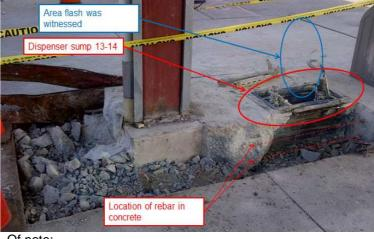
Original JSA had been completed, however 'hot work' was not identified as a relevant critical procedure
