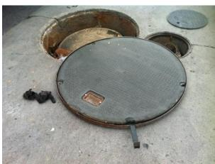
A technician was removing a submersible sump cover plate. The cover plate handle was damaged and the worker was using a prybar to separate the cover plate from the metal sump support ring. The support ring became dislodged from the sump and pinched his finger between the ring and plate. The force of impact resulted in the dislocation of the workers' finger. After seeking medical attention the worker was unable to return to work for 2 days. This lost time injury could have been prevented.
