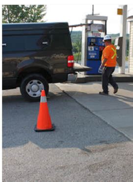
Use vehicle to block work area
