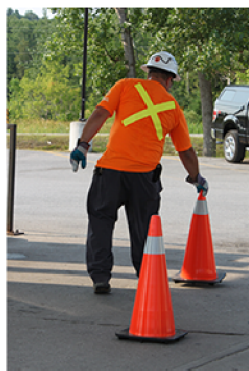
Place cones around work area
