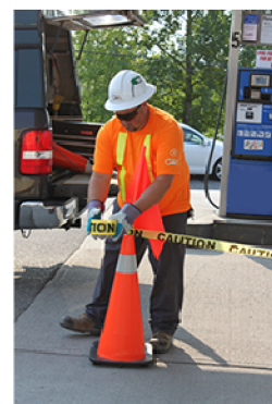
Isolate work area with caution tape
