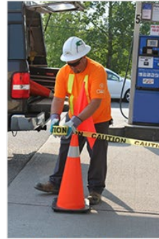
Isolate work area with caution tape
